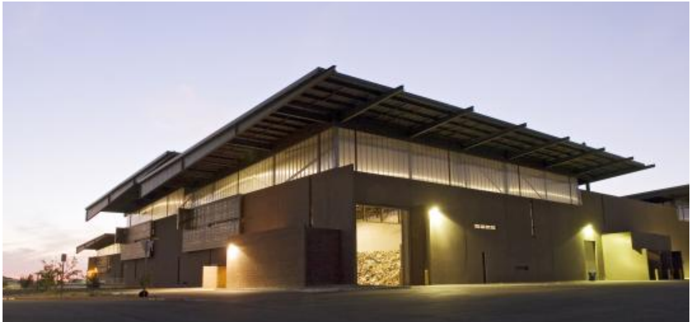
Figure 1.1 RDF Production Facility, Receiving and Processing 432 wet-ton/day MSW
