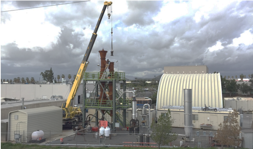
Figure 43: Installing the Detonation Burner on top of the Reformer
