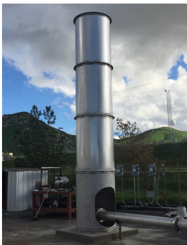
Figure 62: Enclosed-Flare
