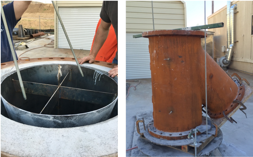
Figure 35: Casting Reactor Sections with Internal Mold
