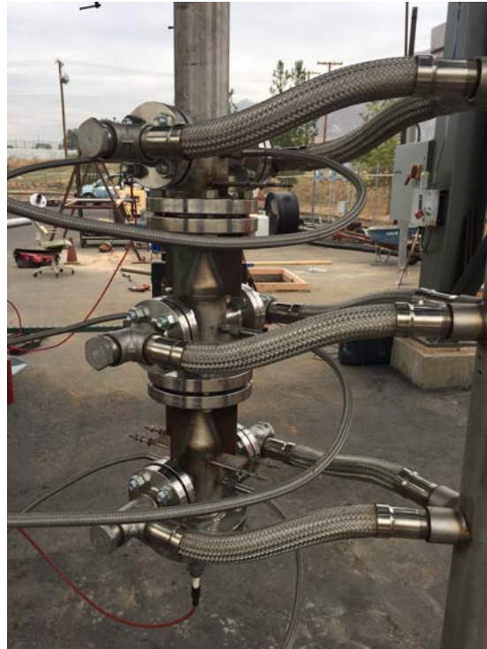
Figure-15. Three-stage prototype installation
